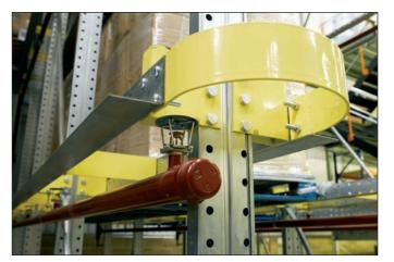
The drive-in racking consists of two blocks of 12 bays, both five levels high and six deep. A very intense sprinkler system has been specified throughout the entire warehouse due to the stringent insurance requirements. As a consequence, some bespoke features were designed into the drive-in racking to maximise storage whilst protecting the sprinkler heads from the pallets as they are driven in and out.
